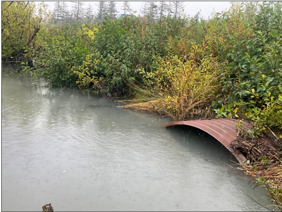
Figure 3.—Twin culvert inlets.
